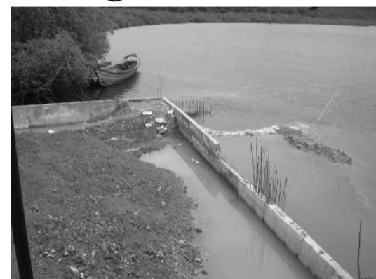
Pic shows fish landing centre under construction at Uttara, Middle Andaman
