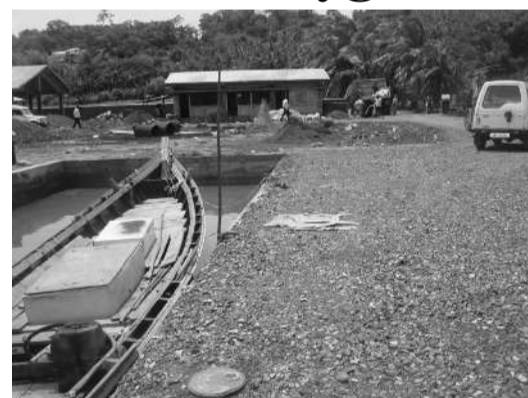
Pic shows Fish landing centre under construction at Guptapara
