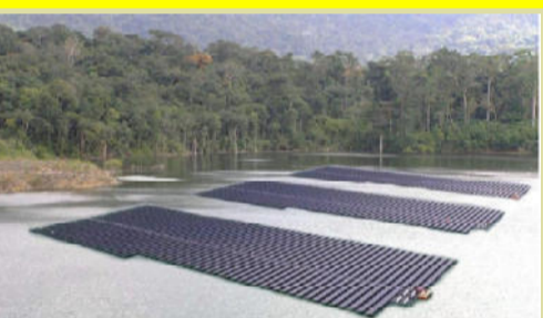
batteries) at Diglipur on Kalpong reservoir in developer mode.
