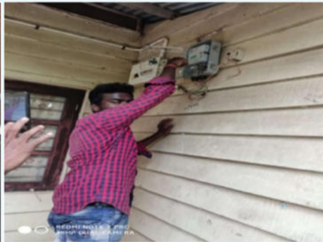
Official of EESL installing Smart Meter at a residence at Tsunami Shelter, Chouldari.
