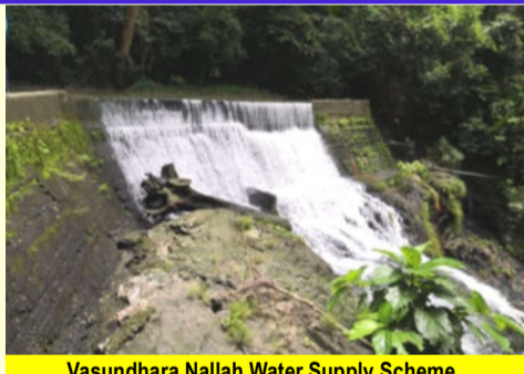
Vasundhara Nallah Water Supply Scheme, Humphreygunj
