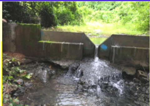
Mini Dam Site at Sippighat
