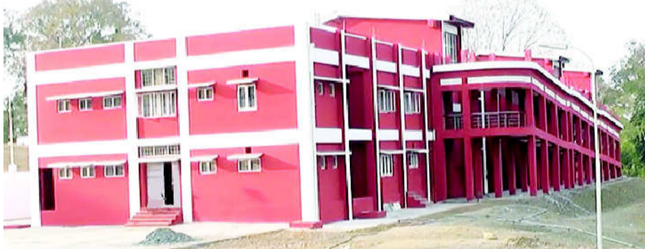
The newly inaugurated District Court Building at Lucknow Village, Mayabunder
