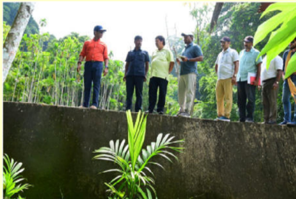
Chief Secretary inspects Check Dam
