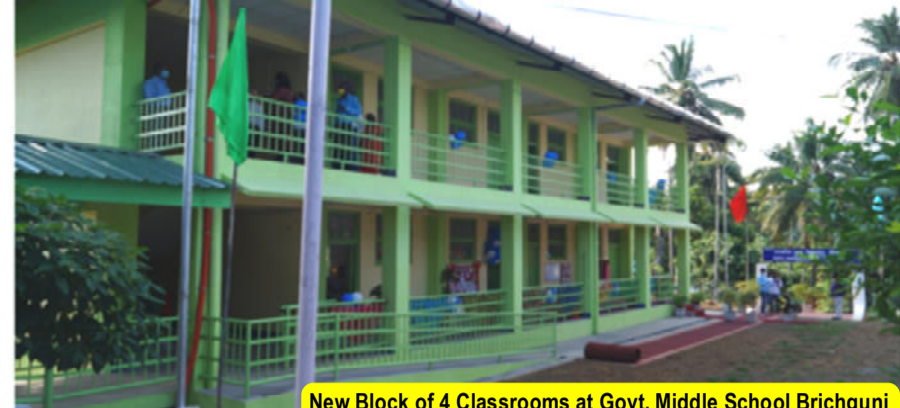
New Block of 4 Classrooms at Govt. Middle School Brichgunj
