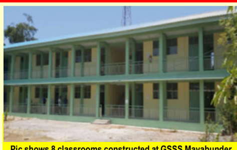
Pic shows 8 classrooms constructed at GSSS Mayabunder
