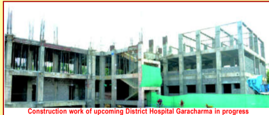
Construction work of upcoming District Hospital Garacharma in progress
