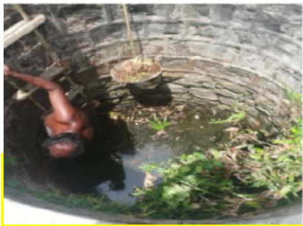
Well cleaned/ rejuvenated at Ward No.22
